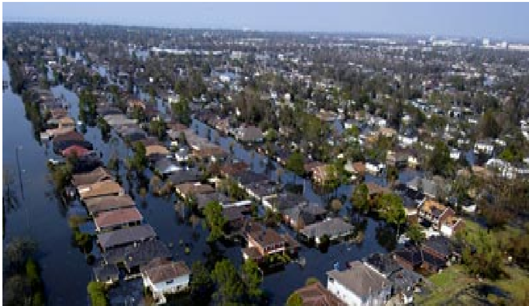
Fig.2 The Flood: Hurricane Katrina's most devastating damage was caused by flooding
